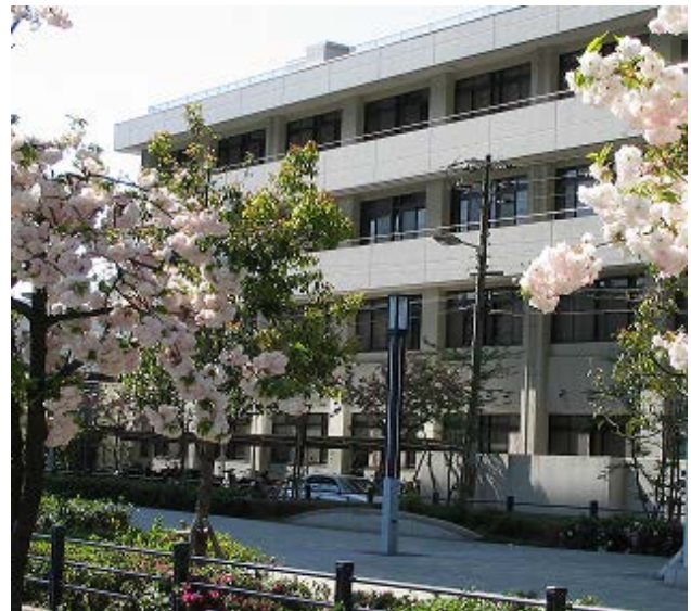
Fig. 11: The first department of Biomedical Engineering in Japan.
